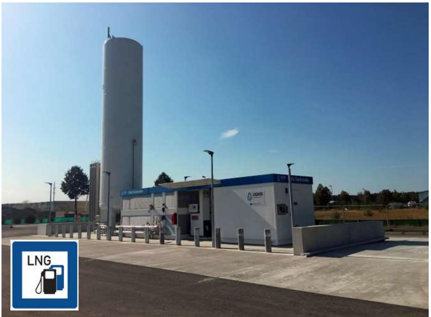
For installing LNG on existing plot, for instance fuelling station, Cryonorm offers design with LNG tank, pump and saturation vaporizer on a skid – required plot area less than 20 m<sup>2</sup>.
