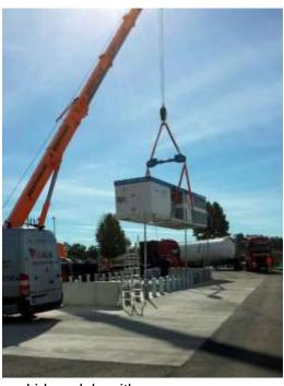
Dispensers, pump and control system are installed inside the skid module with a maximum of two LNG dispensers or one LNG and one CNG dispenser. This design is the perfect solution for green field stations.
